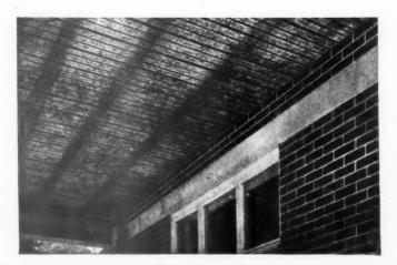
Above right. Hy-Rib sheets in position ready to receive concrete slab. Tubular scaffold may be used for supporting Hy-Rib if timber is not available.
