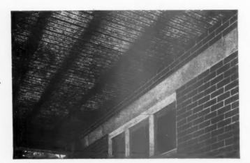
Above right. Hy-Rib sheets in position ready to receive concrete slab. Tubular scaffold may be used for supporting Hy-Rib if timber is not available.
