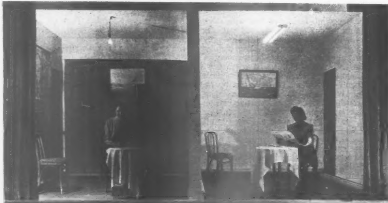
One of the demonstrations used to illustrate Dr. C. C. Paterson's talk at the ELMA lunch reported on this page. On the left is a carbon filament lamp, and on the right two 2 ft. warm tinted fluorescent lamps using the same amount of current.
