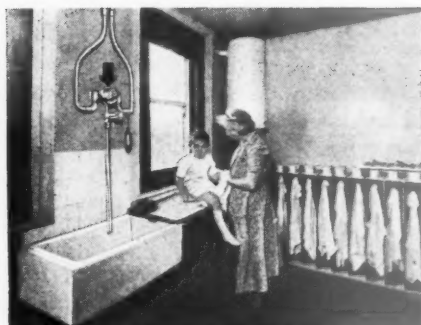
Leonard Thermostatic Mixing Valve serving sink.
