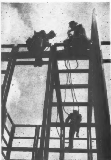
The Braithwaite houses at Hendon under construction. Two sections of the steel frame are being bolted together. See Astragal's note.
