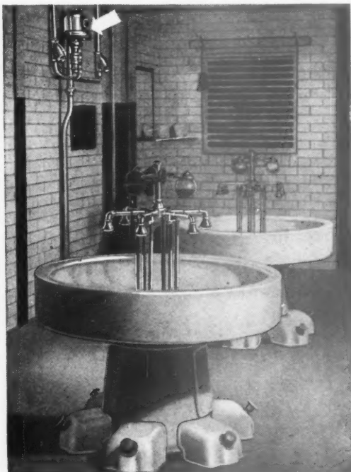
Leonard-Thermostatic Hot and Cold Water Mixing Valve serving ablution fountain for factory workers. Courtesy of the M.G. Car Co., Ltd.
