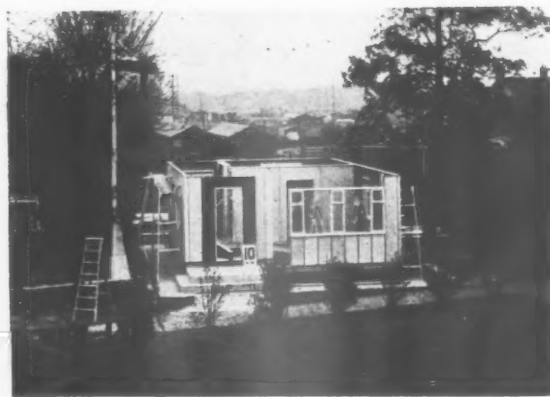
10 a.m., May 2. First floor walls going up.
