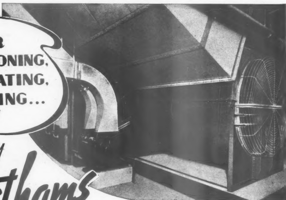
One of several 9ft. diameter Multivane Fans installed by Cheethams of Oldham for the Air Conditioning of one of the largest Aircraft Factories in England.
