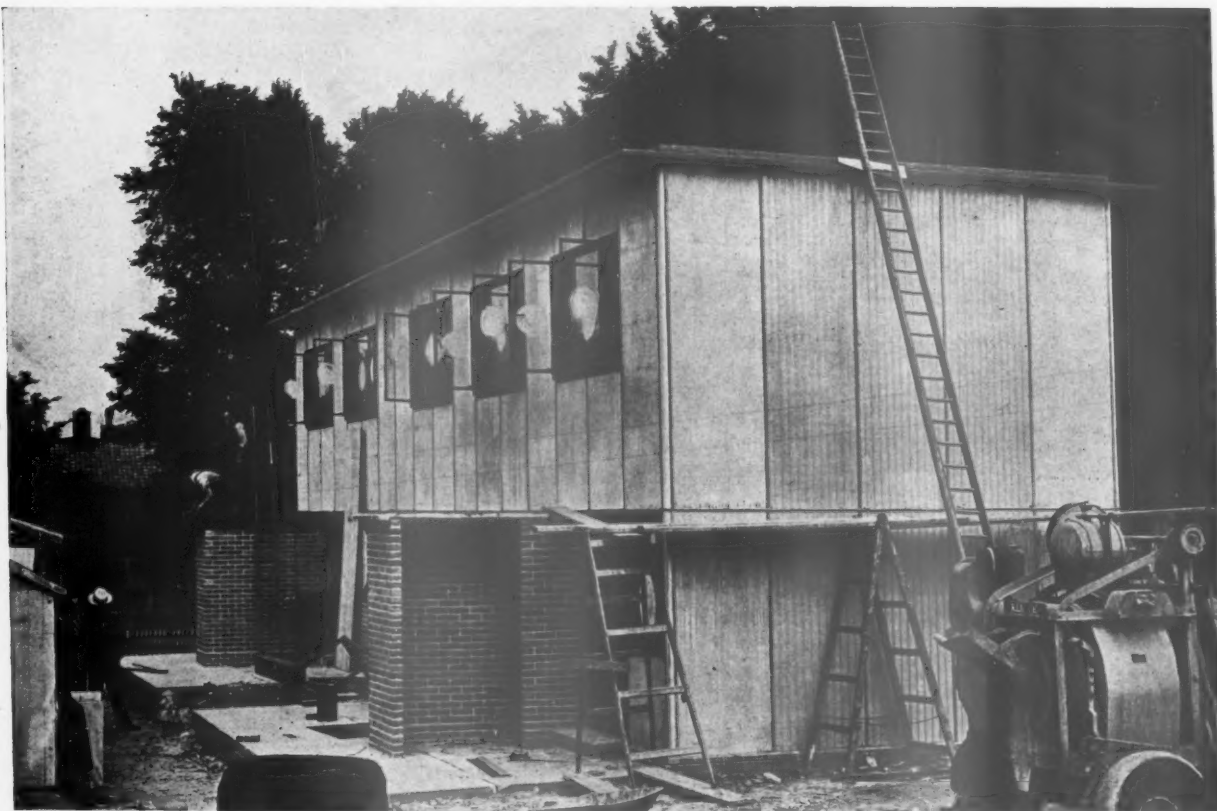
Above, the job nears completion. Note the brickwork on the garden elevation. Brick is a possible cladding material as well as local stone. Below, ground and first floor plans of the houses at Hendon designed by F. R. S. Yorke. The grid dimension used throughout is 3 ft. 2 in.
