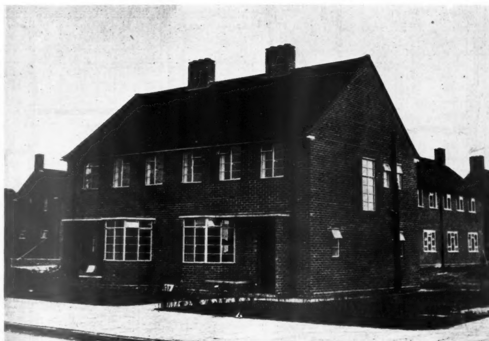
1, 2, 3 Top. house No. 1 of no fines concrete with a rendered external finish. Nos. 2 and 6 are identical in appearance. Above, house No. 3 with bays and brick finish. No. 10 is similar.
