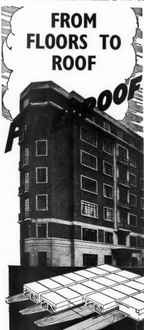
The SMITH TWO-WAY reinforced fireprooffloor can be employed immediately for any flooring or roofing requirement. It is constructed with standardised pre-cast hollow concrete blocks.
