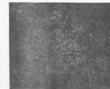
Cracking of paint on interior work, due to improper sequence of coats, necessitating removal before repainting. The illustrations are from The Painting of Buildings . (See No. 1660.)
