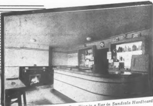
Panelling to a Bar in Sundeala Hardboard.
