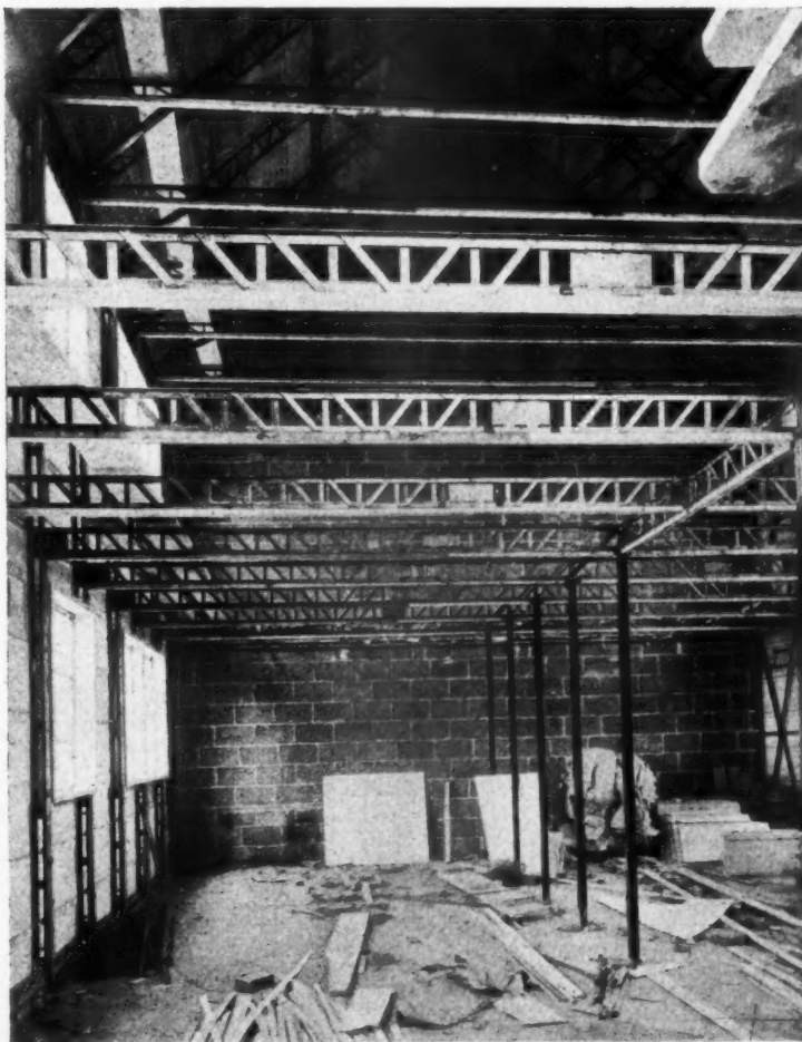
One of the most interesting of the MOW demonstration houses at Northolt under construction—the flatted dwelling designed to reduce site labour, of a light steel frame of the same patented type as that used in the Birmingham house. The cladding is of 2-in. concrete slabs, the walls being insulated with glass wool and faced internally with wall boarding.
