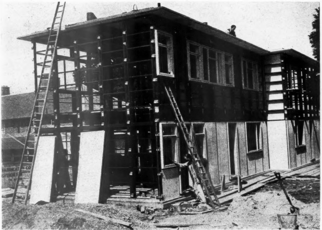
The Braithwaite pair of demonstration houses of steel unit frame under construction on the LCC Watling Estate.
