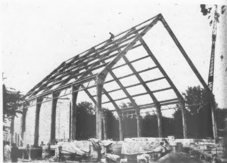
A welded design for a church in the USA having a 45^\circ roof pitch with no lateral bracing. See No. 1805.
