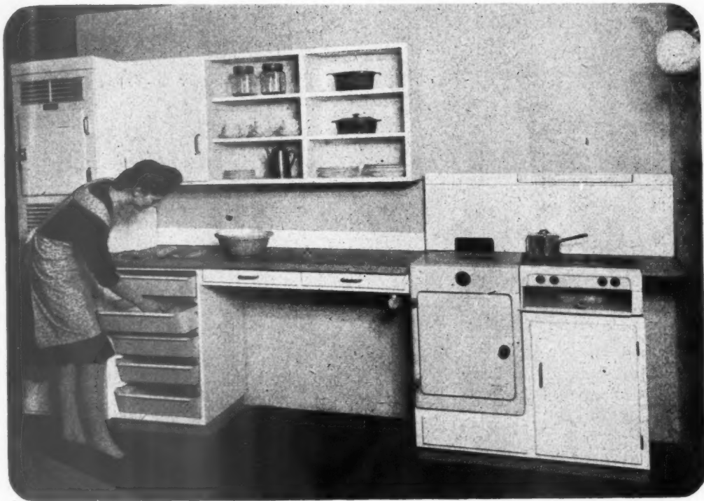
Left, combined kitchen units which can be mass-produced in a variety of materials suitable for existing houses. New units can be added from time to time as needed. The units here are timber, except for the vegetable drawers of enamelled steel. Below, a mural by F.H.K. Henrion.
