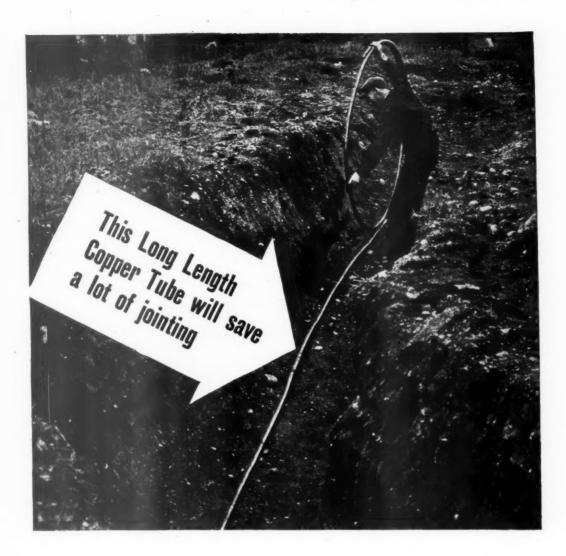
Installation costs of domestic water supply services will be much reduced by the use of "KUTERLON" Long Length Copper Tube which is now supplied in coil form in lengths up to 60 ft. Annealing or the use of mechanical bending appliances are not necessary. Bending can be done by hand,
