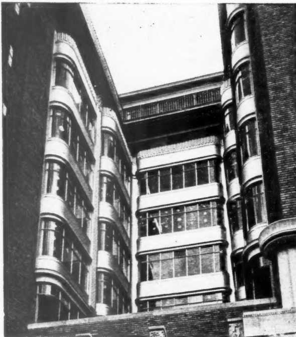
Above : Cast Iron Panels in the bays of the new Adelphi Building on the Embankment, London.
