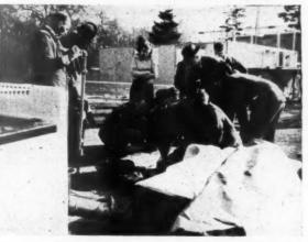
4 The first roof panel is being hoisted into position. The roof is of twelve wedge-shaped units, about 4 ft. by 12 ft., with two smaller units for the porch roof. Underside is faced with wallboard, and the top surface is flat asbestos sheet covered with three layers of single ply roofing felt. The roof is lined with a blanket type of insulating material.
