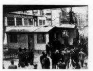
Top, the first section of the house being manoeuvred into position on the brick foundations. Below, from left to right, progress photographs showing the remaining three sections being moved into position.
