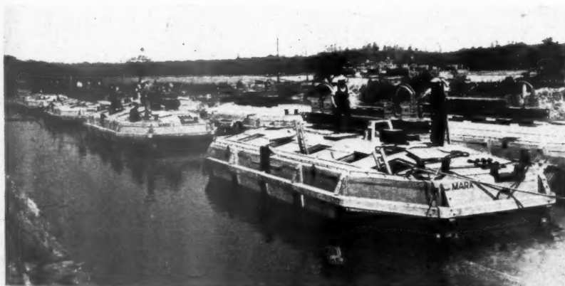
Top, one of the timber shuttles used on the Mulberry Harbour for laying pontoon anchors at great speed. Below, a number of reinforced concrete pontoons, or Beetles, after launching and before they were towed across to the French coast. See Astragal's note.
