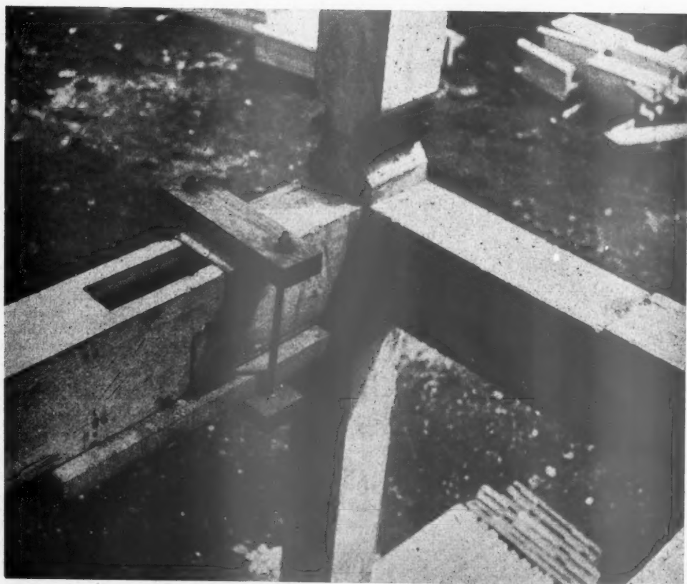
Top, base bonders in position showing an angle post with its metal connector at the joint. Left, a close-up showing the connections of members at the first floor level. The joint on the left is ready for its concrete infilling.
