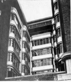
Above : Cast Iron. Panels in the bays of the new Adelphi Building on the Embankment, London. Architects: Messrs. Collcutt & Hamp, FF.R.I.B.A. Contractors : Gee Walker & Slater.
