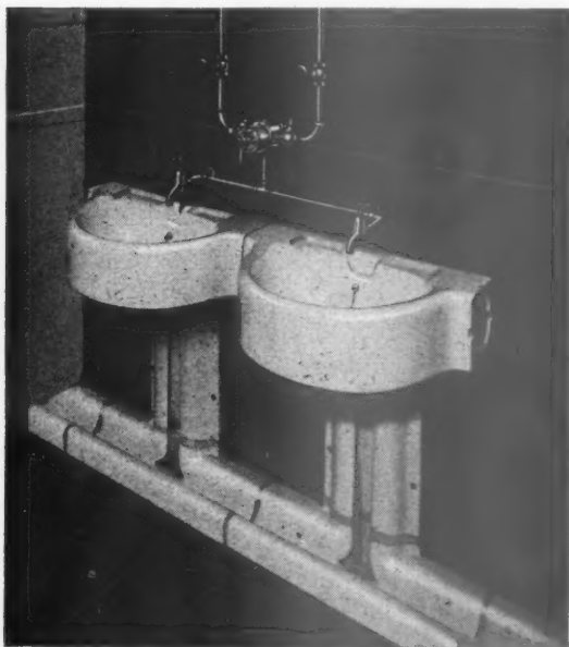
Leonard-Thermostatic hot and cold Water Mixing Valve serving wash-basins.
