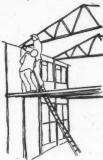
Bolting of roof truss.
