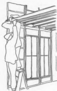
Fixing of floor joist.
