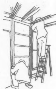
Fixing of cleats between wall units and bolts to floor joists.
