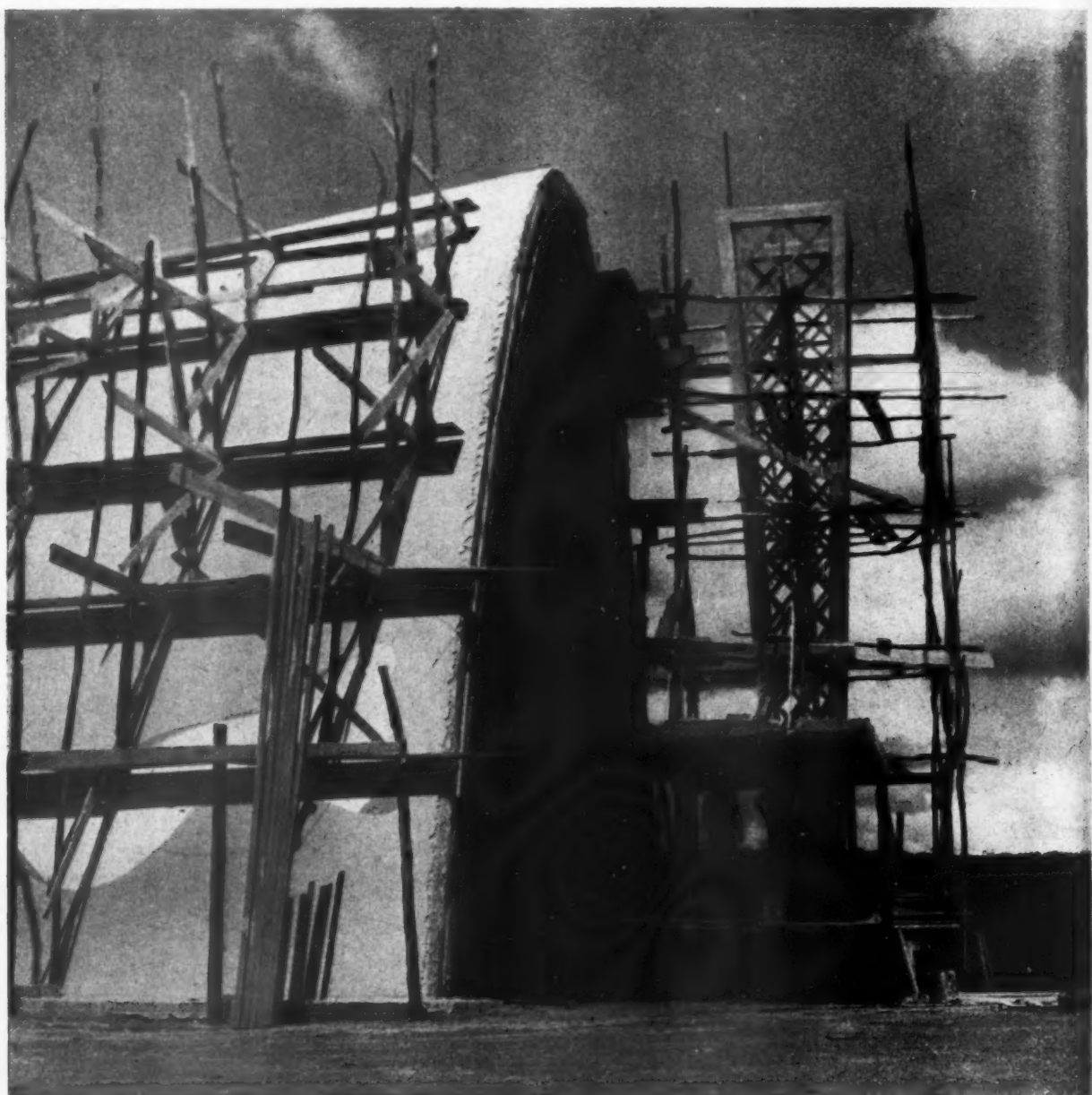
Above, a church, at Pampulha, Belo Horizonte, designed by Oscar Niemeyer, now nearing completion; it is of reinforced concrete parabolic arch construction. Below sketch of the front elevation, which faces a river; on the right is the bell tower.
