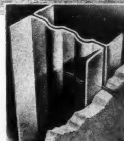
Wall sections of light-gauge steel for Navy houses, Jacksonville, Fla., were placed by hand. These 16-ga. sections contain patented nailing grooves (right) for attaching wall material to steel framing. See No. 2346.
