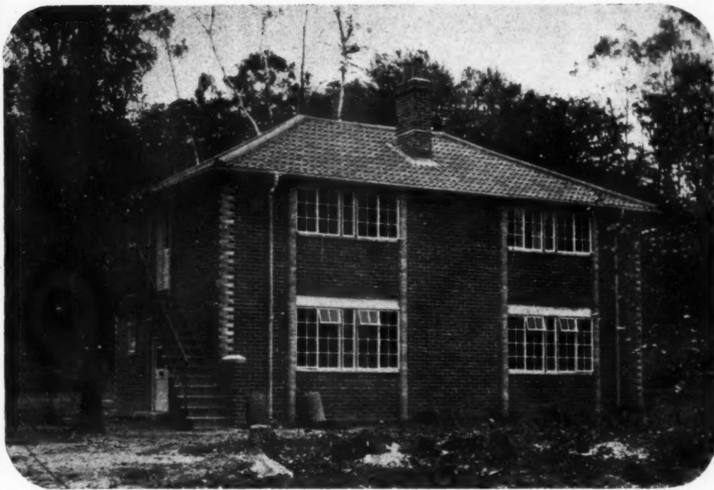
Left, the completed house. Below left, diagram showing main principle of construction of concrete pier blocks, holding reinforcing rods, and 4\frac{1}{2} in. brick non-load-bearing screen walls.
