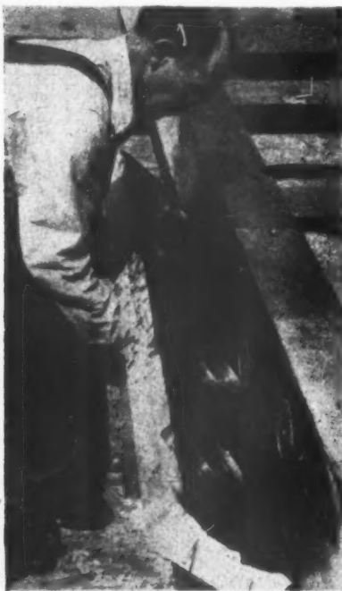
Split rings, which in recent years have become standard practice in the USA for timber connections, carry the load, the bolts merely holding parts together. See No. 2397.
