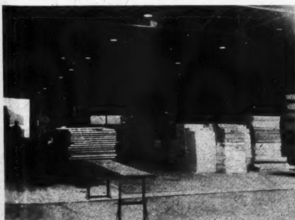
At a large assembly plant for prefabricated houses at Elstow, near Bedford. Here all the essential parts are collected and dispatched by lorries to the sites where the houses are to be built. Each lorry is loaded piece by piece and moves off bearing all the parts of a prefabricated house.
