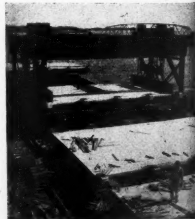
The deck of a Virginia highway bridge is precast at a central yard in 40 ft. long sections. See No. 2417.
