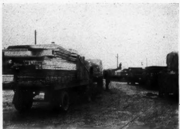
At a large assembly plant for prefabricated houses at Elstow, near Bedford. Here all the essential parts are collected and dispatched by lorries to the sites where the houses are to be built. Each lorry is loaded piece by piece and moves off bearing all the parts of a prefabricated house.
