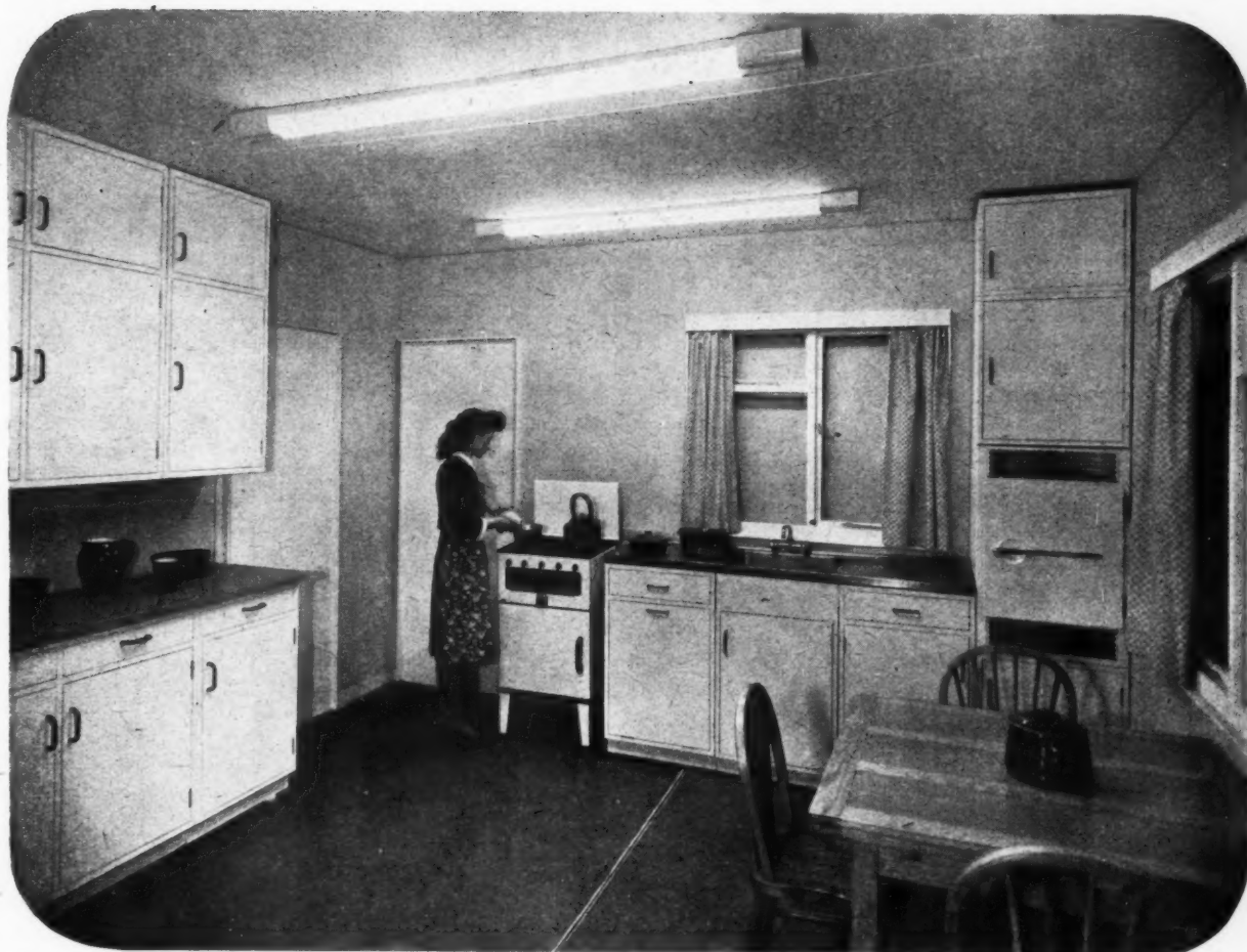
An all gas kitchen designed by Sir Percy Thomas, President of the RIBA. It has standard size fittings and is planned to cut out unnecessary movements through correct working sequence. The sink is of stainless steel. A refrigerator is incorporated on the right at eye level. Hot water is provided by a back boiler installed with the living-room gas-ignited coke fire, supplemented by a gas water heater for summer use.
