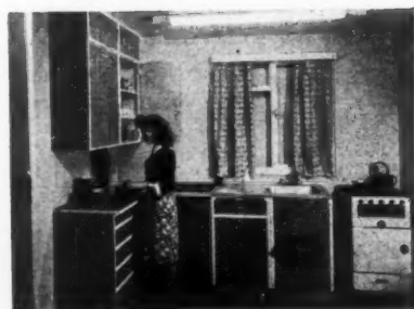
Above, another of the gas operated kitchens designed for Government houses. The fittings are standard size, as they are in the design on the right. Here the sink has a garbage bin below it; the storage cupboard is conveniently over the working surface.
