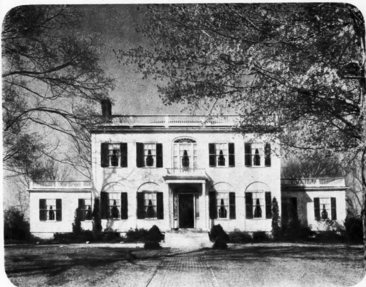
The Headmaster's House, Phillips Academy, Andover, Mass. A frame house built in 1811, and designed by Bullfinch (1763-1844). The lower wings have lapped boarding exterior, but the main block has a close boarded covering, with filled joints.
