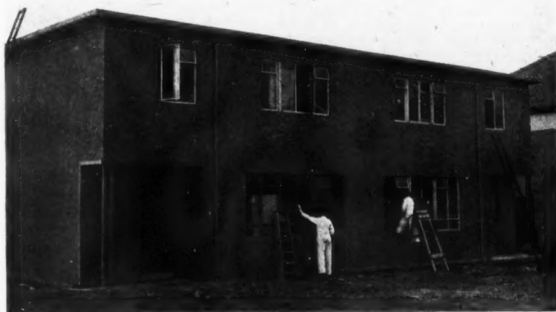
Painters lining off the window frames and putting the finishing touches to the first Weir steel house erected at Knightswood, Glasgow.
