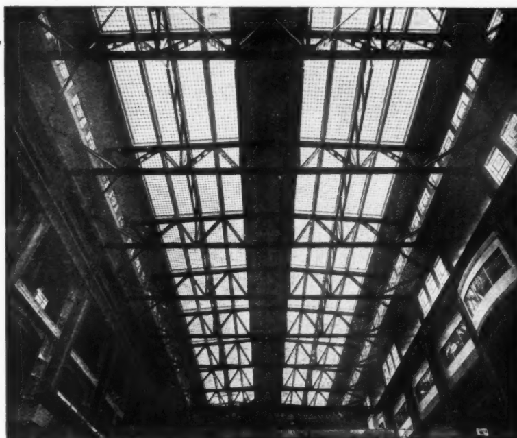
The illustration is of the roof to the turbine house at Fulham Power Station where many thousands of sq. ft. of GLAS-CRETE constructions were installed. The construction shown is double glazed in order to minimise the risk of condensation which is a vital point in connection with electrical machinery.
