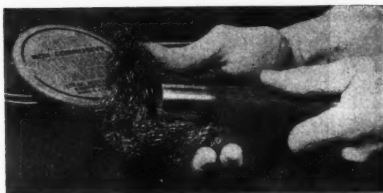
The copper tube and fitting, to be joined, must be cleaned with steel wool leaving both surfaces bright.
