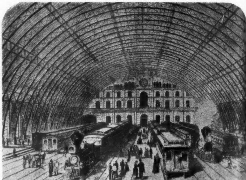
First Grand Central Station, New York, 1871, which was the largest interior in the USA at that time, being 200 ft. wide and 600 ft. long. Its open-web arched girders, probably imitating those of St. Pancras, are of cast and wrought iron. See No. 2586.
