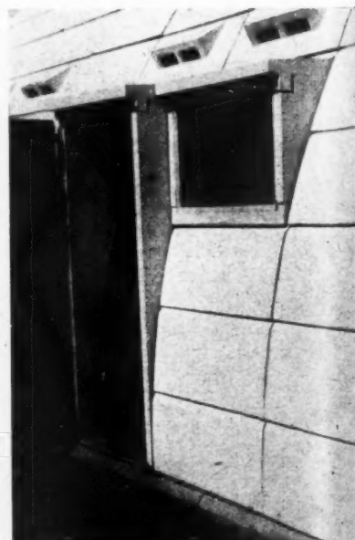
Left, one of the reinforced concrete curved standards in position. Centre, view of interior of wall. Right, close-up showing door and window construction of precast elements, and ventilating slabs; joints are shown without their mortar filling.
