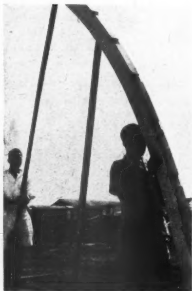
Left, one of the reinforced concrete curved standards in position. Centre, view of interior of wall. Right, close-up showing door and window construction of precast elements, and ventilating slabs; joints are shown without their mortar filling.
