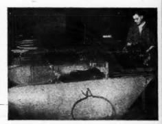
Cutting off the ' cap ' of a hand-blown cylinder.
