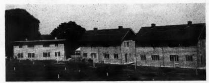
Airey permanent prefabricated houses on the London County Council estate at Ching ford, Essex. Between the prefabricated concrete outer walls and the fibre board lining glass fibre is used for insulation.
