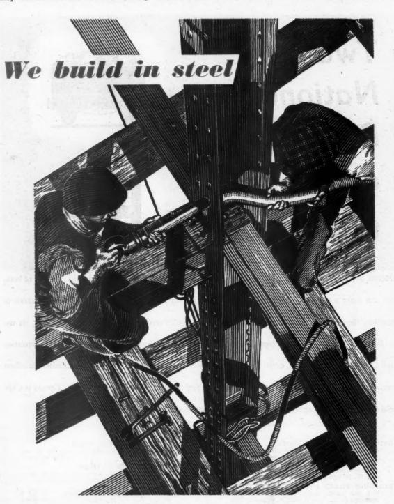
PREFABRICATION is in the air. But there's nothing new about it; the principle has been in operation for many years in the construction of steel frame buildings. Steel units of many kinds are put together (pre-fabricated if you like) by the structural engineers, and arrive at the site ready to go immediately to their planned positions. It all makes for economy and speed
