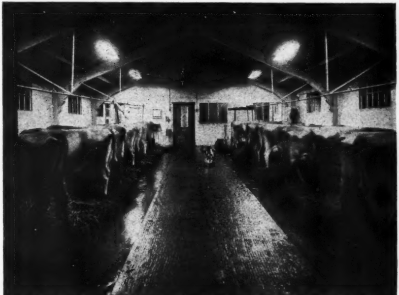
Cowshed with standings for twenty-four, built by Sidney L. Hill, Ltd., for C. D. Notley's pedigree herd of TT. and Attested Jerseys at Firethorn Farm, Ewhurst. The lighting is by six 80 watt Atlas fluorescent tubes and the photograph was taken by fast exposure without any additional lighting.
