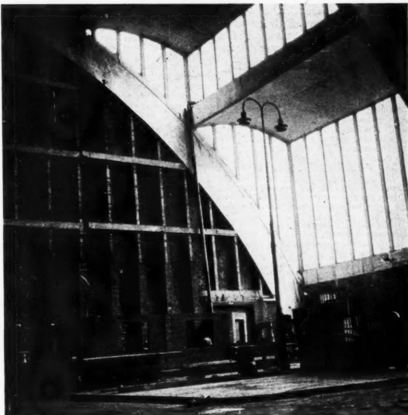
An example of German shell concrete construction, the Slaughter House at Kiel. The photographs were taken by the BIOS team which visited Germany. See No. 2781.
