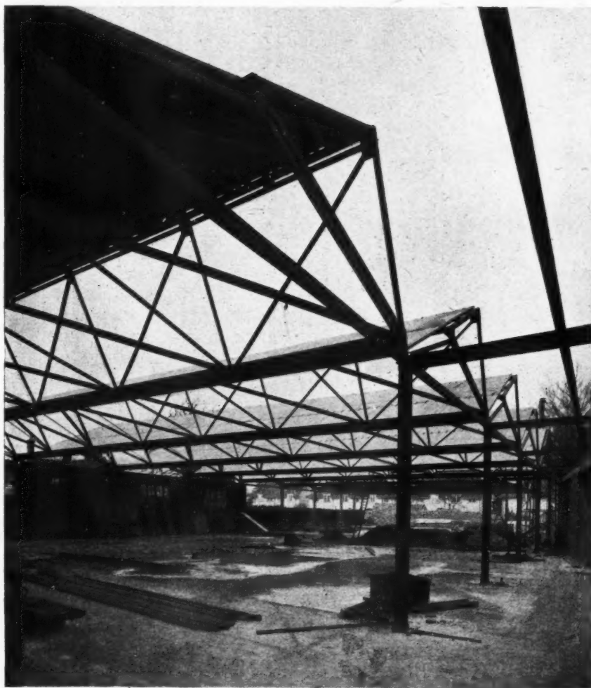
Above, another view of the factory during construction, showing close-up of the end of a bay. Below, diagram of a space frame unit as hoisted.
