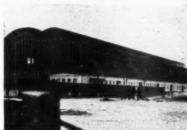
An example of German shell concrete construction, the Slaughter House at Kiel. The photographs were taken by the BIOS team which visited Germany. See No. 2781.
