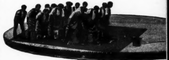
"Swimming the Plate" in the Disc Grinding Process
