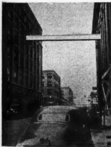
Moving day at a Portland, Oregon, crockery store which Astragal describes above. Left, the plywood bridge spanning across the street from the old building to the new. Right, the interior of the bridge through which the goods were rolled.
