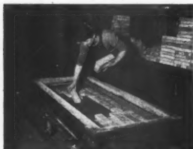
1. Laying brickettes for a wall unit in a steel mould.
