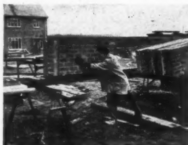
5. The unit, steam cured for speed of setting, is rolled on to the site on a conveyor.
