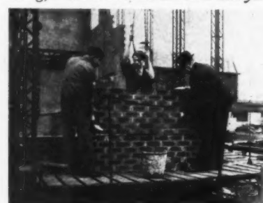
6. The prefabricated wall unit being laid in a prototype house.
