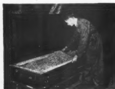
3. Filling the mould with lightweight concrete.
