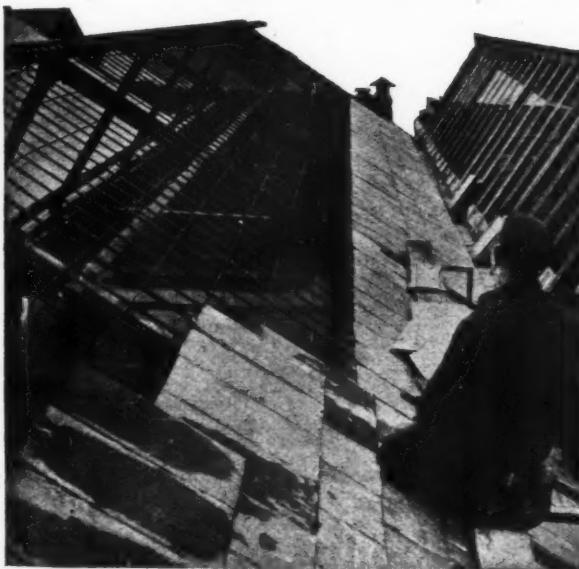
Two views of the roof of a weaving shed in Lancashire. The contract was for approximately 1500 sq. yds. of roofing consisting of eleven bays each approximately 190 ft. long. (Roofing Contractors: The Manchester Slate Co. Ltd.)
