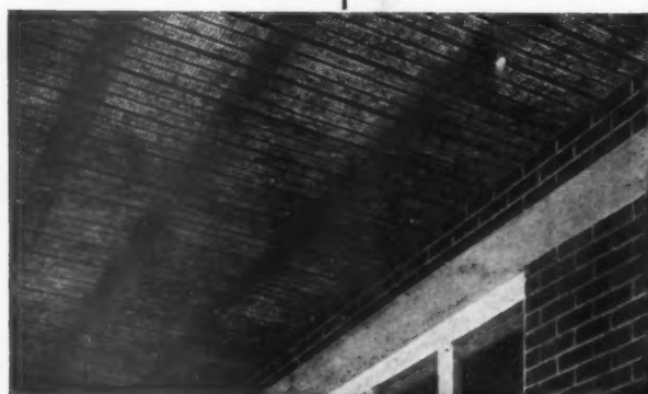
NOTE: READY KEYED SOFFIT FOR CEILING FINISH
