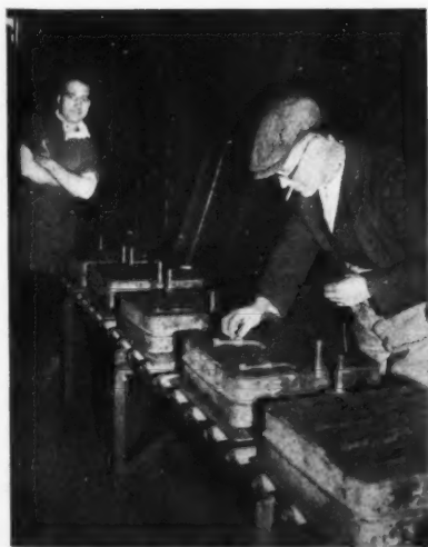
The Royal Ordnance factories in many parts of the country are turning their efforts to peaceful channels. Above, casting taps at Woolwich Arsenal.
