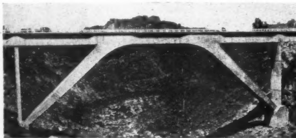
A 264 ft. span reinforced concrete rigid frame aqueduct crossing an Oregon canyon. See No. 2867.
