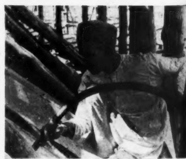
The Taj Mahal has recently been cleaned and repaired, for which purpose a strange scaffolding mainly of bamboos was erected round the dome. A general view is shown on page 140. Top, inside the spiral ramp formed by the scaffolding. Below left, a new block of marble being inserted to repair a damaged rib in the dome. Centre, mixing the special mortar. Right, a workman discharges cement under pressure into a crevice.
