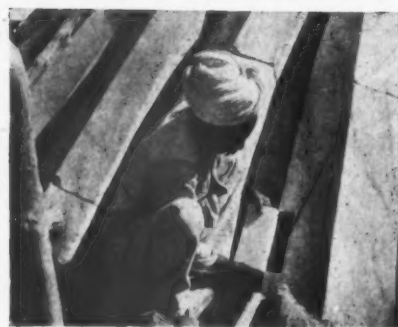
The Taj Mahal has recently been cleaned and repaired, for which purpose a strange scaffolding mainly of bamboos was erected round the dome. A general view is shown on page 140. Top, inside the spiral ramp formed by the scaffolding. Below left, a new block of marble being inserted to repair a damaged rib in the dome. Centre, mixing the special mortar. Right, a workman discharges cement under pressure into a crevice.
