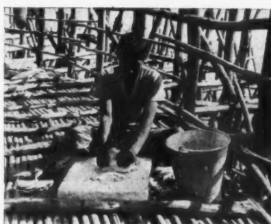
The Taj Mahal has recently been cleaned and repaired, for which purpose a strange scaffolding mainly of bamboos was erected round the dome. A general view is shown on page 140. Top, inside the spiral ramp formed by the scaffolding. Below left, a new block of marble being inserted to repair a damaged rib in the dome. Centre, mixing the special mortar. Right, a workman discharges cement under pressure into a crevice.
