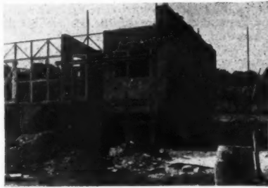
Progress photos showing the timber framings to the external wall to the corridor.
