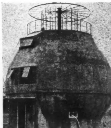
Spherical concrete-and-welded-steel dwelling in USA. The steel ribs are constructed around a large metal cylinder which carries a forced air gas heating and air conditioning unit and acts as a chimney. The flattened roof acts as a glassed-in solarium. See No. 20.10.
