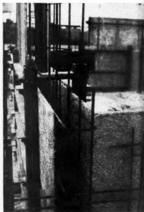
The junction of a transverse wall with an external wall during construction, showing the reinforcement and wood-wool inner lining (used as permanent framework) before concreting.
