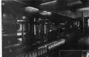
Part of the restaurant installation of Messrs. Debenham and Freebody Ltd., of Wigmore St., W., showing electric and steam cooking apparatus. Equipment is of special finish with stainless steel boiling pans, counters, sinks, etc. Ventilation hoodwork of anodised aluminium.
