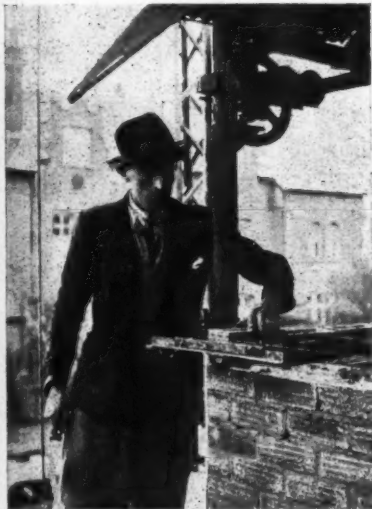
A corner post of the Warry steel framed jig.
