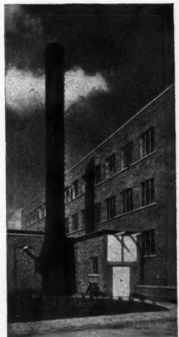
Above, a general view of the building which has red brick walls and reinforced concrete and steel frame structure; the loading bay can be seen on the extreme right. Left, the canteen on the top floor. Below, the west elevation and boiler house.
