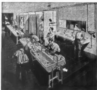
Leonard Valves serving a range of wash-hand basins, range of showers and washing-troughs.
