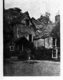
1940, and June, 1942. On stripping the stucco work, fine oak halftimbering was revealed, on to which lathing had been nailed to form a key for the plaster work. Two small oak window frames were also uncovered, which have been reglazed. All the woodwork has now been exposed.
