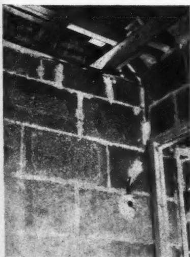
The flexible conduit can be run in the corner between partitions and on the underside of ceiling joists.
