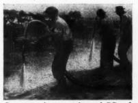
Cement guns in use on damaged RC roof. See 20.39.
